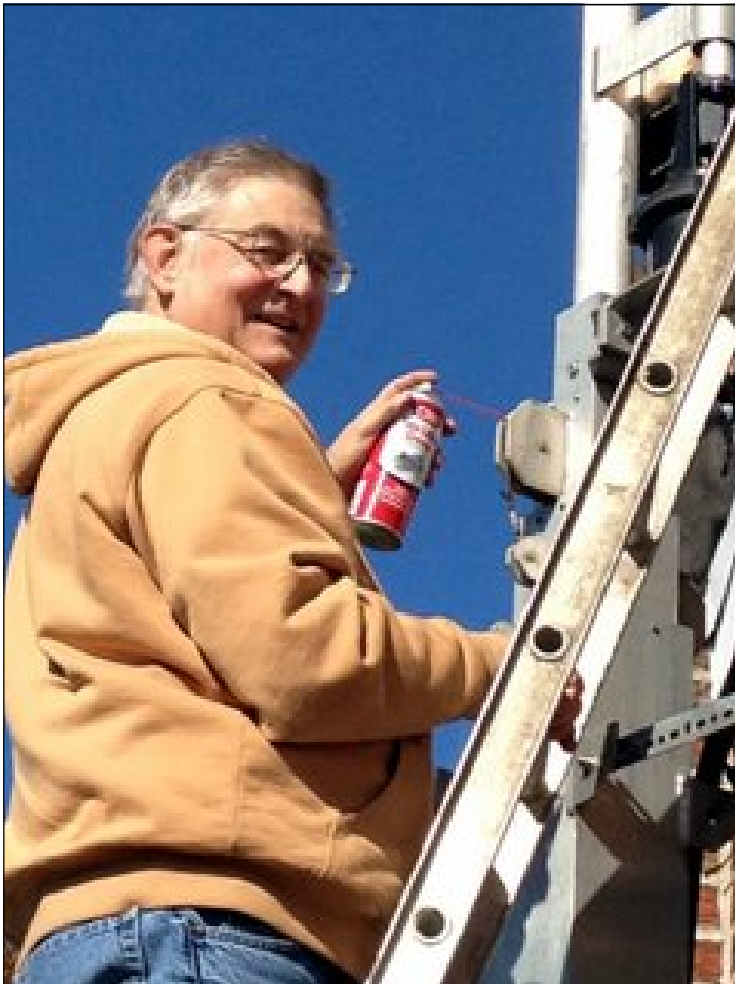
KA3WXV does some pulley maintenance on EI's tower
