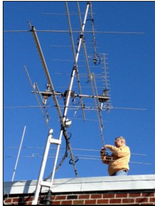
KA3WXV fixes the 2304 feedline connections
